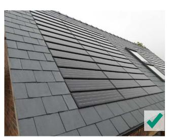
**Figure 127:** Integrated solar panels on slate roof.
