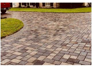
**Figure 133:** A good example of permeable paver (Source: https://www.paverconnection.com/testimonial/hedwig-village-permeable-driveway-and-patio-upgrade/)
