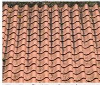
Figure 45: Red pantile roof
