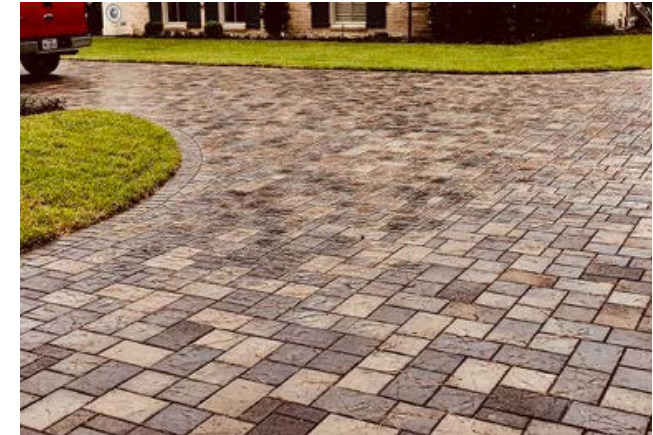
Figure 133: A good example of permeable paver (Source: https://www.paverconnection.com/testimonial/hedwig-village-permeable-driveway-and-patio-upgrade/ )
